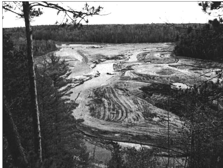
Figure 5. Boardman River Dam Removal Project Site (source: author)
